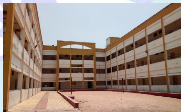
Boys Hostel at SSR
